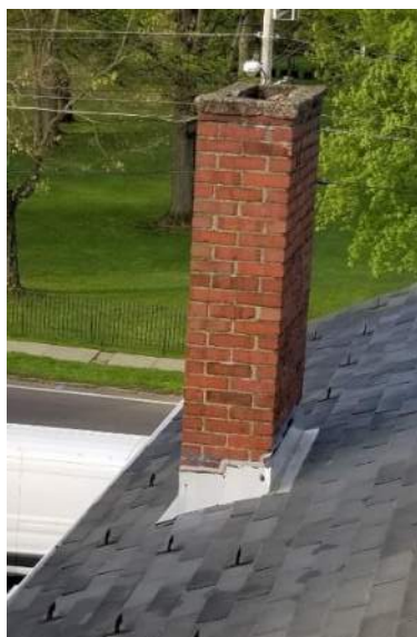
Figure 7: Existing Chimney Flashing.
