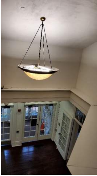
Photograph 28: Horn/Strobe and Pull Station.
