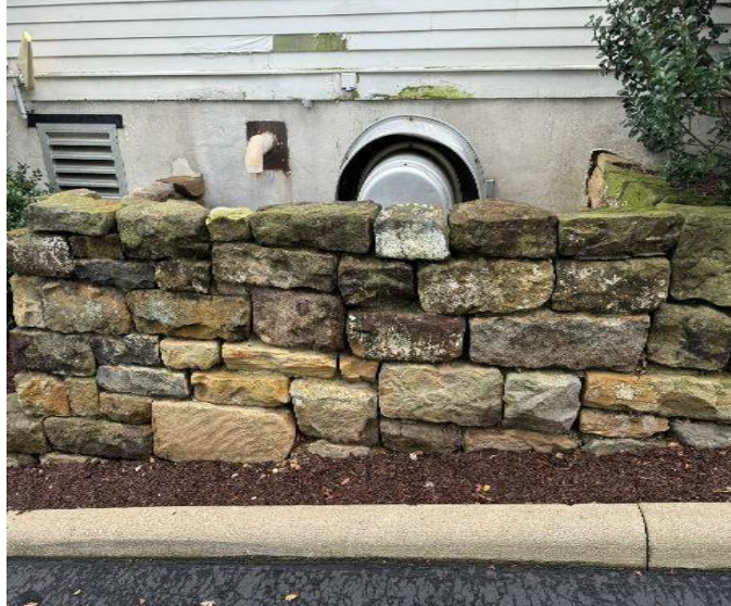
Photograph 18: Kitchen EF Discharge.
