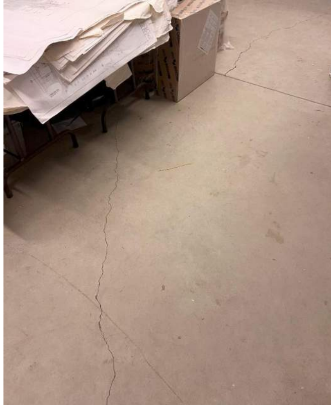
Figure 3: Concrete Slab in Electrical Room.
