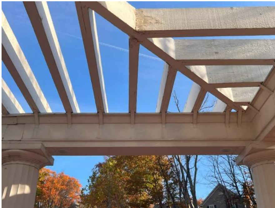
Figure 7: Metal-strap connections on pergola assembly near parking lot.
