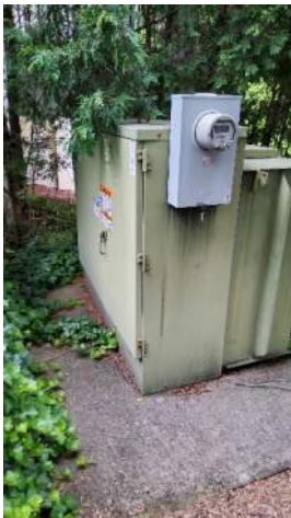
Photograph 20: Utility Transformer.
