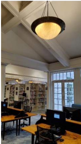
Photograph 24: Reading Area Lighting.
