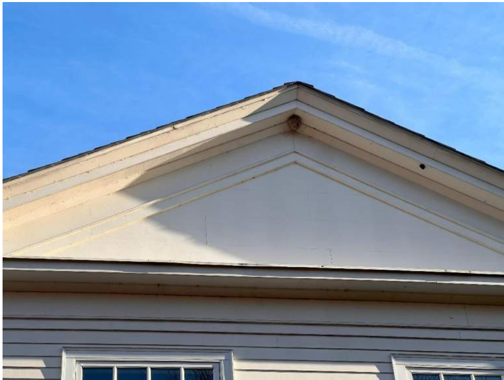
Figure 4a: Pediment on the Northwest corner of the building.
