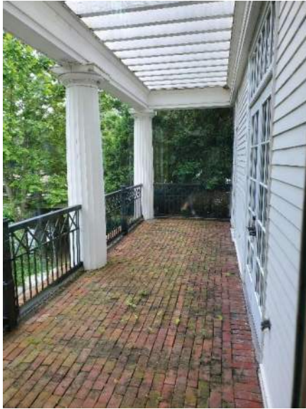
Photograph 20: Standard photography of the south balcony looking west.
