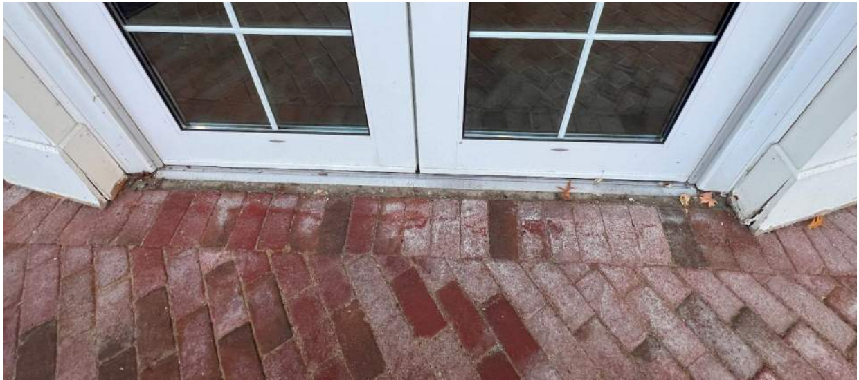
Figure 8: Door sill at East entrance. Note both pilaster bases.
