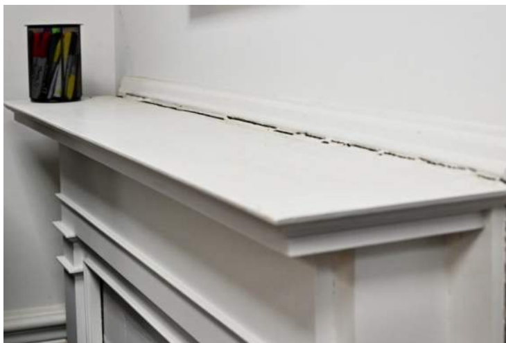
Figure 6: Fireplace located on the second floor.
