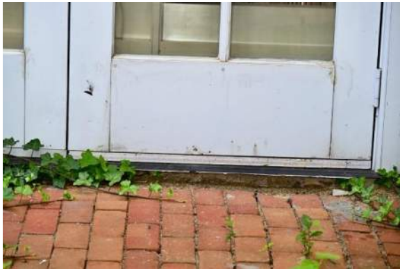
Figure 1: Pavers are recessed below the door at this patio location.
