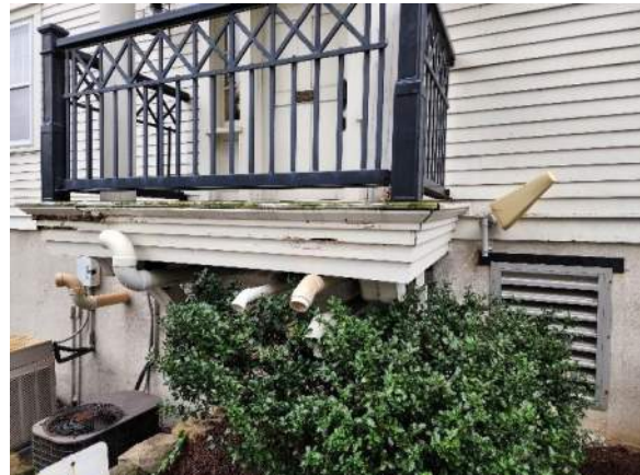
Photograph 12: Close up of the north side balcony.
