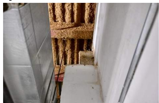
Figure 4: Looking up at the floor beam.
