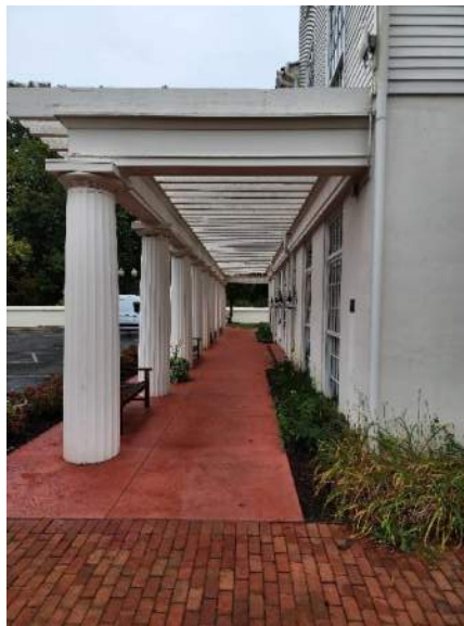
Photograph 6: East sidewalk slopes toward building.
