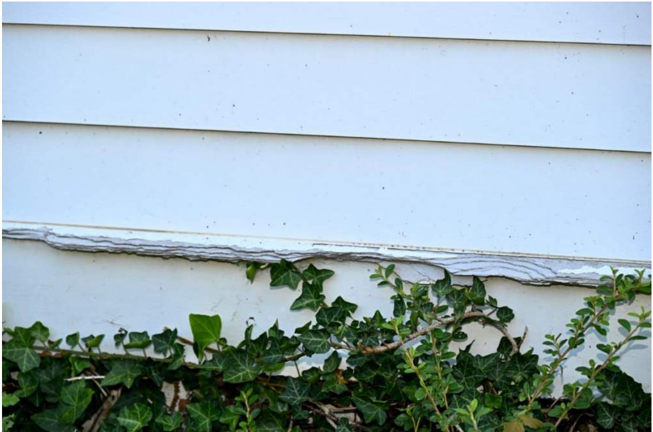
Figure 2: Wood trim on the North Elevation of Dorm. Bldg.
