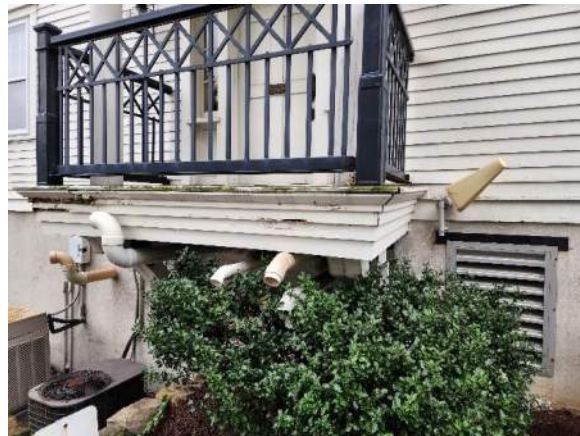
Photograph 12: Close up of the north side balcony.
