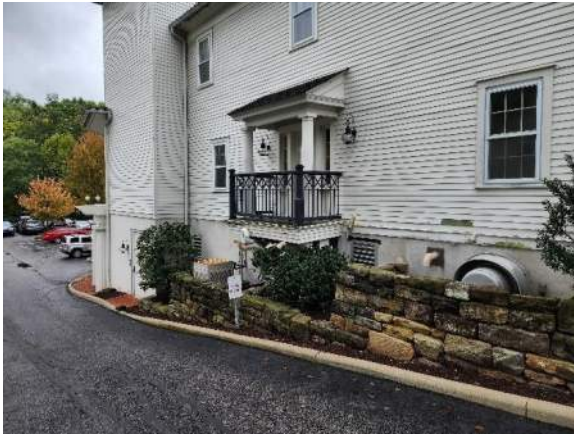
Photograph 11: Standard photograph of the north side balcony.
