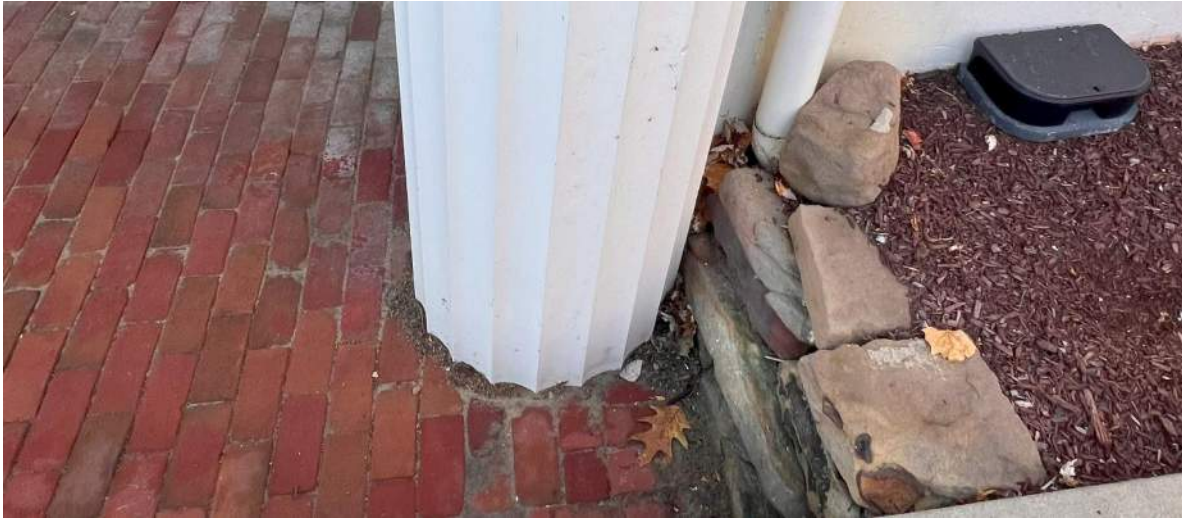
Figure 1: Column base at East entrance.
