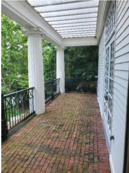
Photograph 13: Standard photograph of the south balcony looking west.
