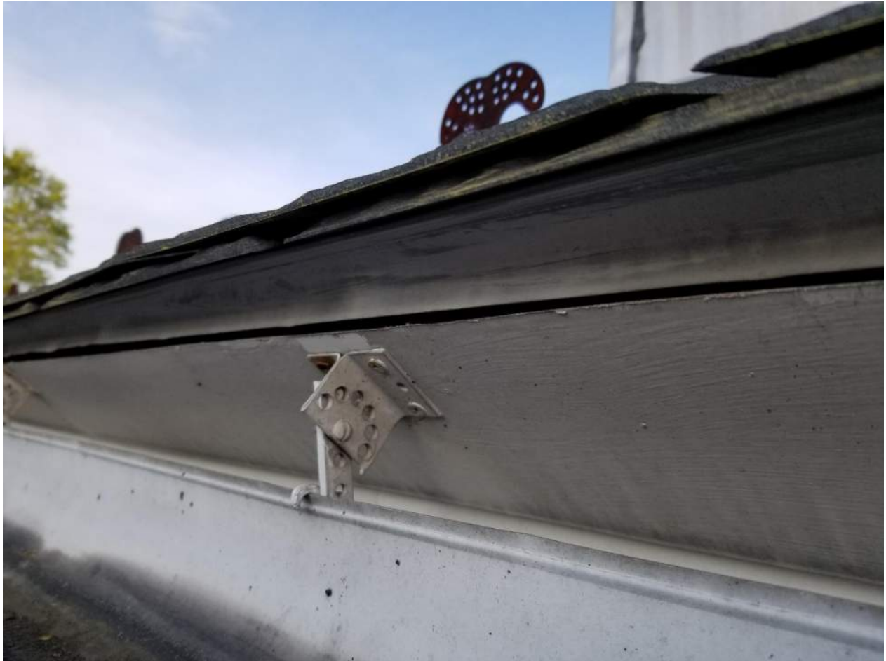
Figure 1: Closeup of gutter configuration.
