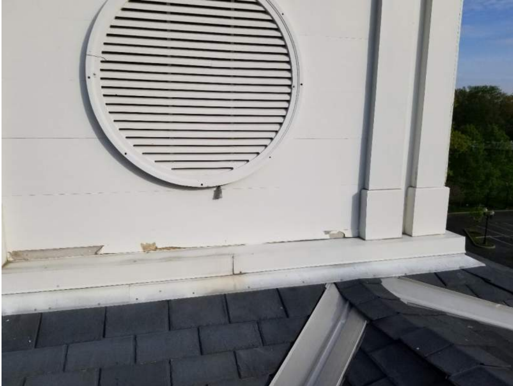
Figure 13: View of cupola occupied near the Dormitory Bldg.
