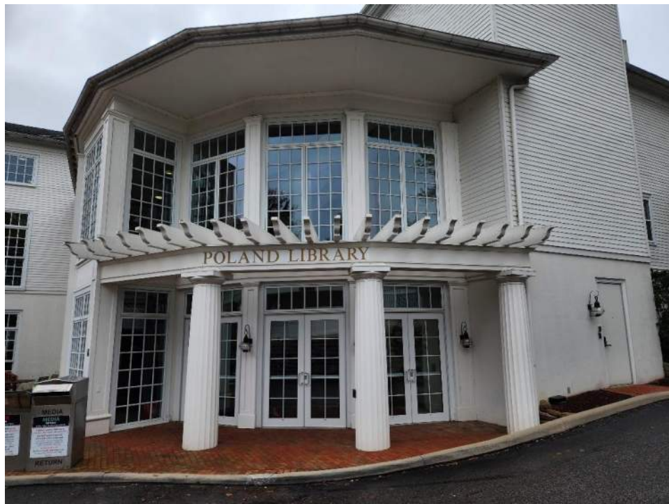
Photograph 1: Main Entrance to the Poland Library looking south.
