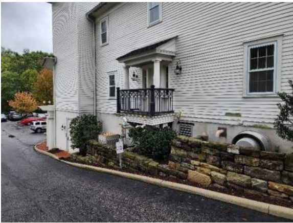
Photograph 11: Standard photography of the north side balcony.
