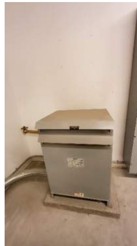
Photograph 22: Step-Down Transformer.
