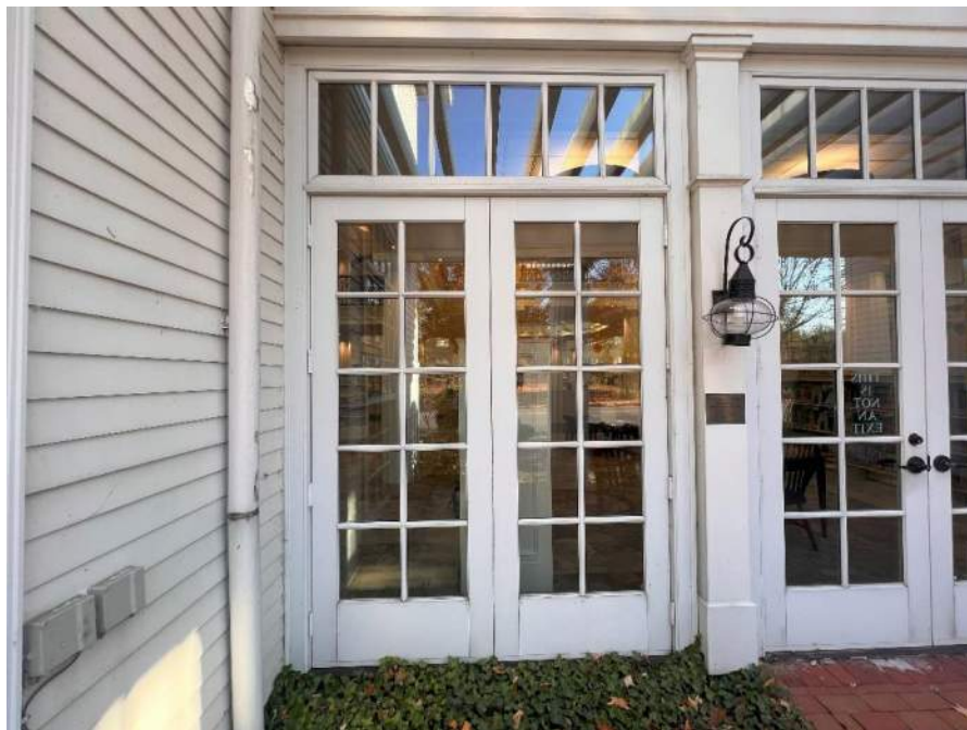
Figure 11: Fixed double doors front profile (Northeast patio).
