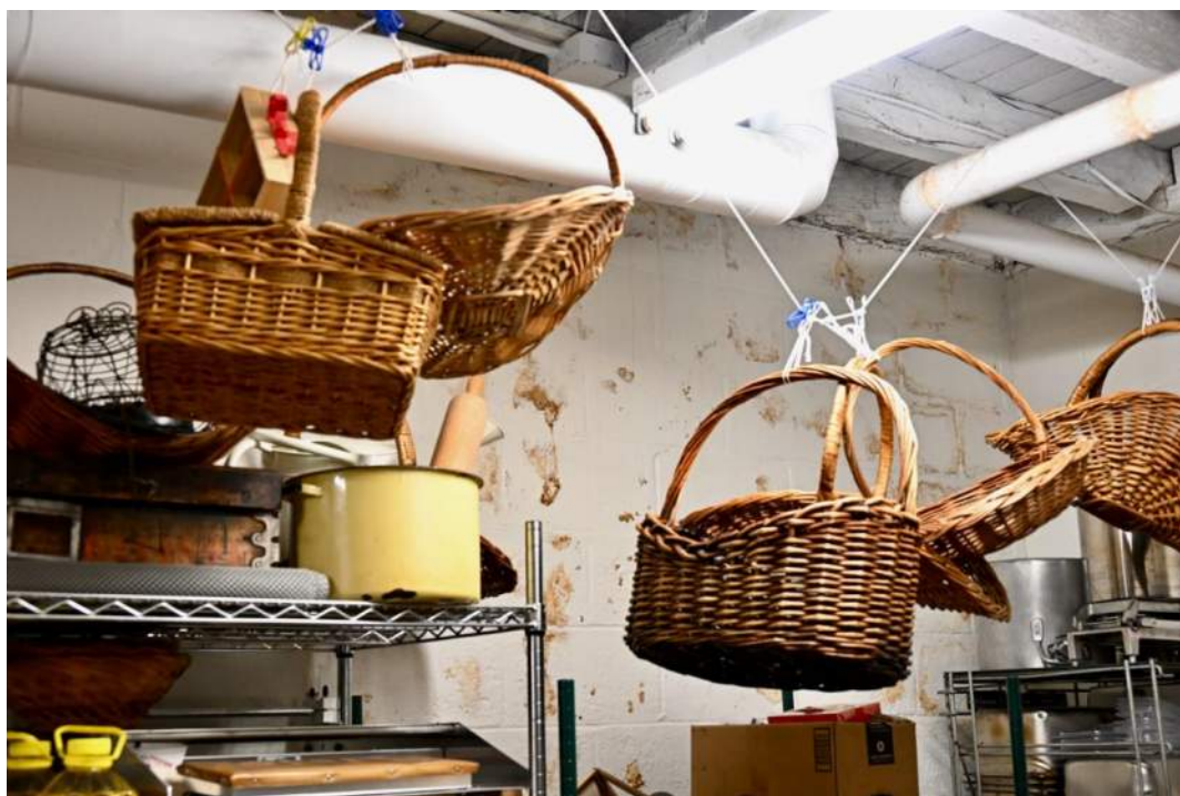
Figure 4: Discoloration of foundation wall.
