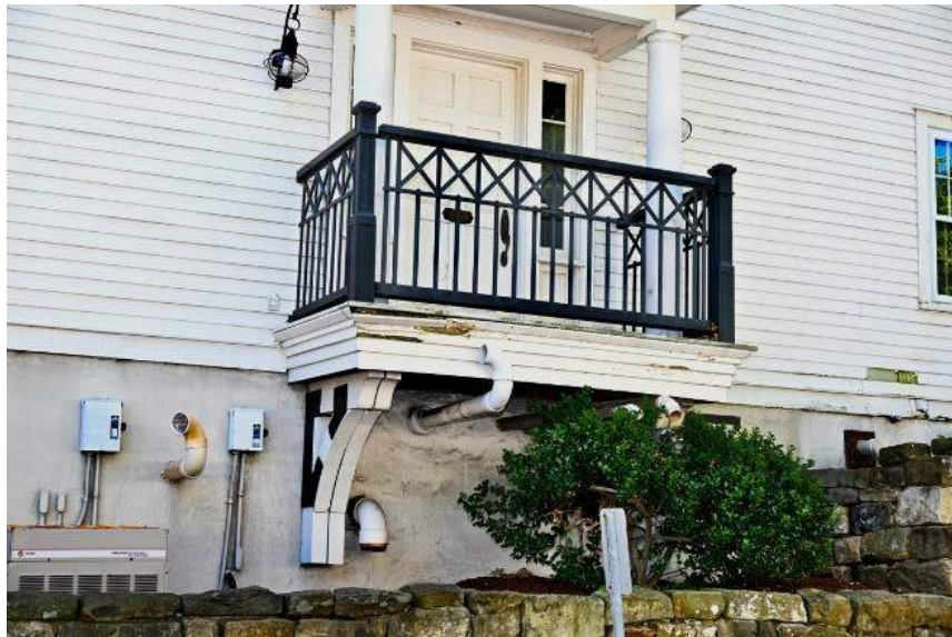
Figure 8: Porch located on exterior wall. Note exhaust location.
