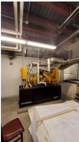
Photograph 23: Standby Generator.
