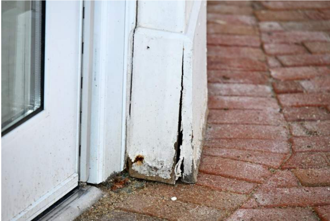
Figure 6: Typical repair of pilaster base at the main entrance.
