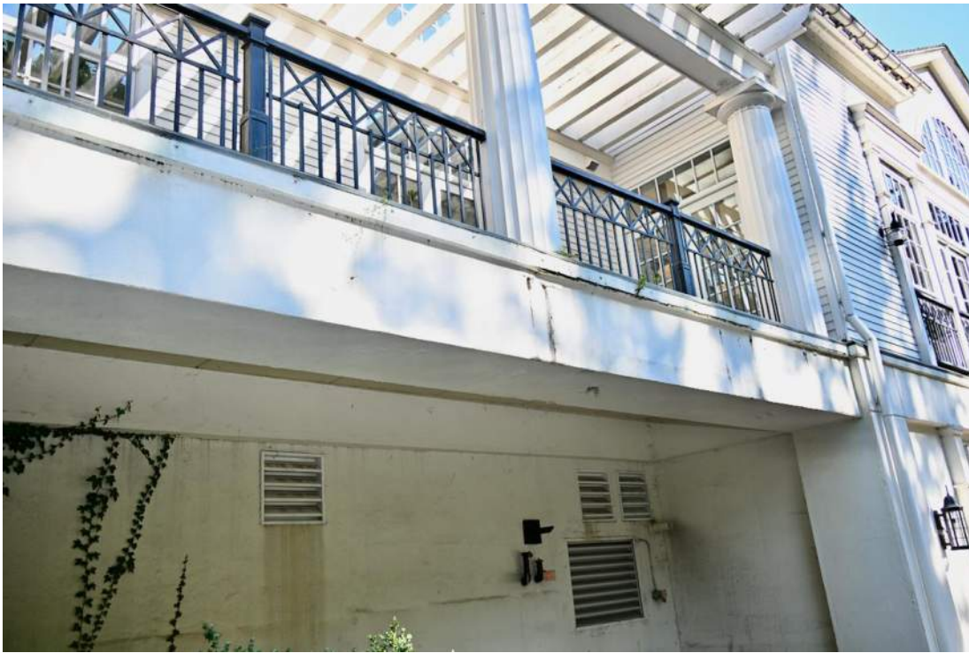
Figure 3: View underneath the main-level balcony.
