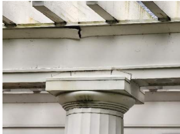
Photograph 10: Close up of the west side southern pergola.
