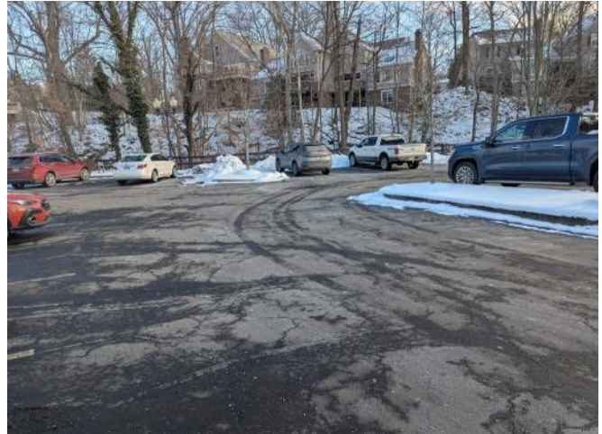
Figure S-3: Parking lot conditions
