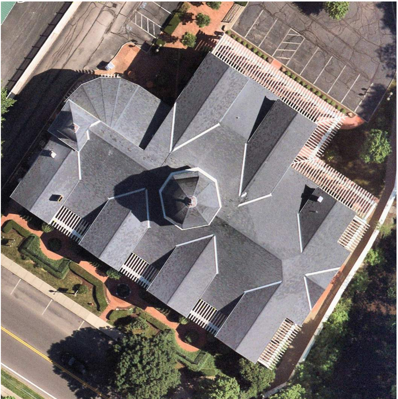
Figure A-5: Roof Aerial
