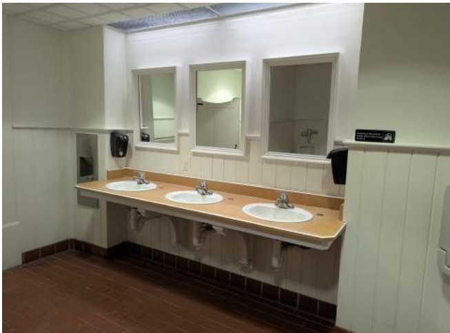
Figure A-14: Men's restroom lavatories
