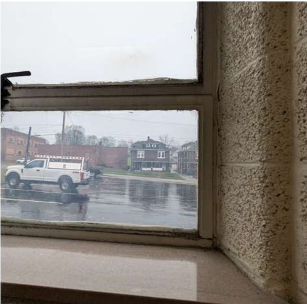
Single pane steel sash windows
