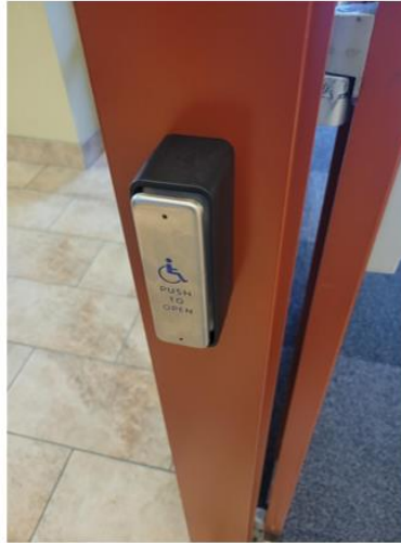
MK – New Door Openers (above and top right)
